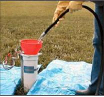
system. These solids can cause clogging of faucet aerators, valves, water solenoids and equipment using filters. Run the water out on the ground until the water runs clear. Additional chlorine solution may need to be added to the well. Do not start recycling water down the well until the water from the hose is clear.
